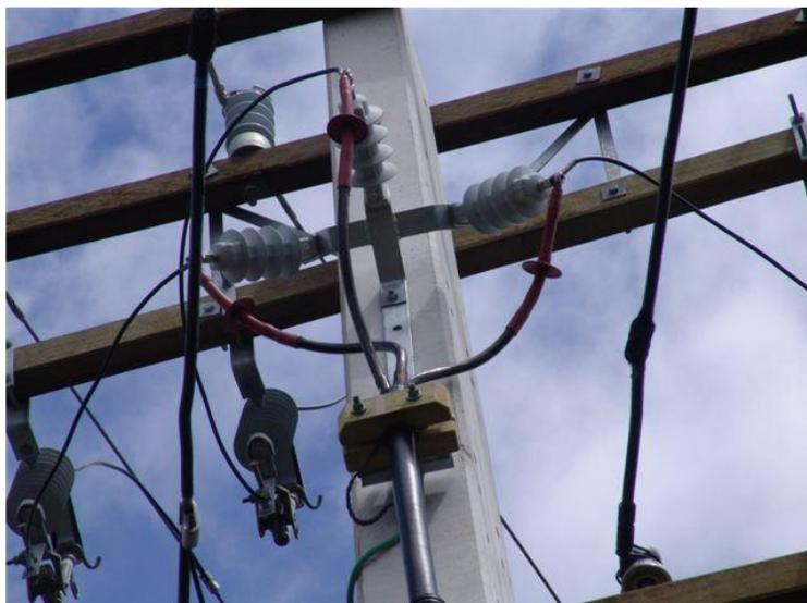
Figure 7: Surge Arrester Crucifix Example
