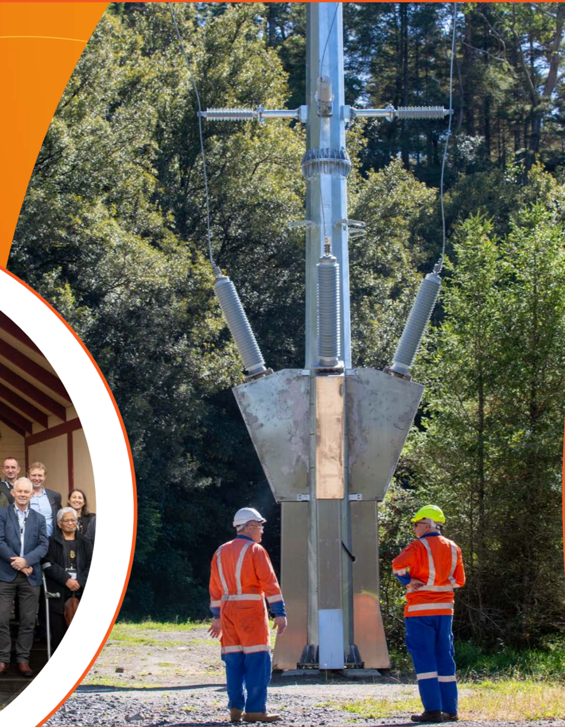
The South Waikato National Grid Connection commissioning event at Mangakaretu marae
