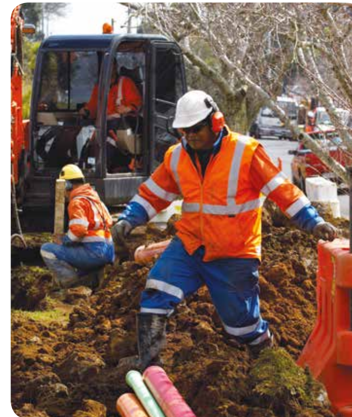
▲ Our crew installing underground cables.
